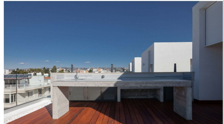
3D Views | Roof Top
